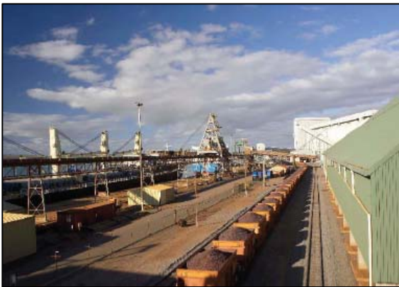
Figure 14: Rail track approaching Berth 4
