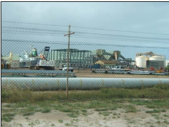
Figure 17: Berth 5 under construction
