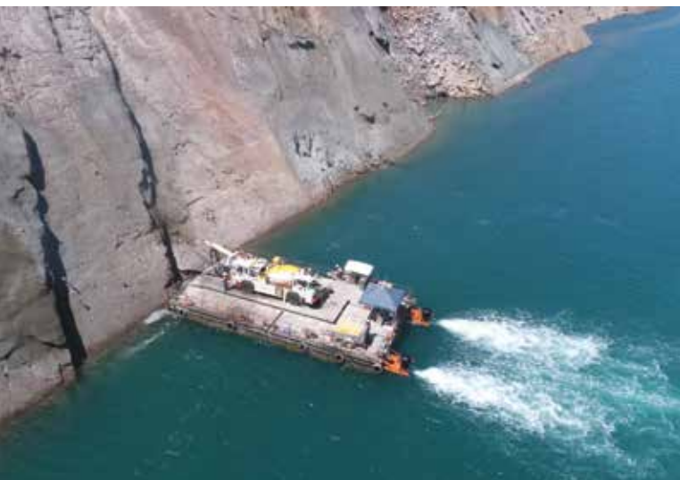
Barges were used to support installation of a seepage barrier to the Koolan Island seawall.
