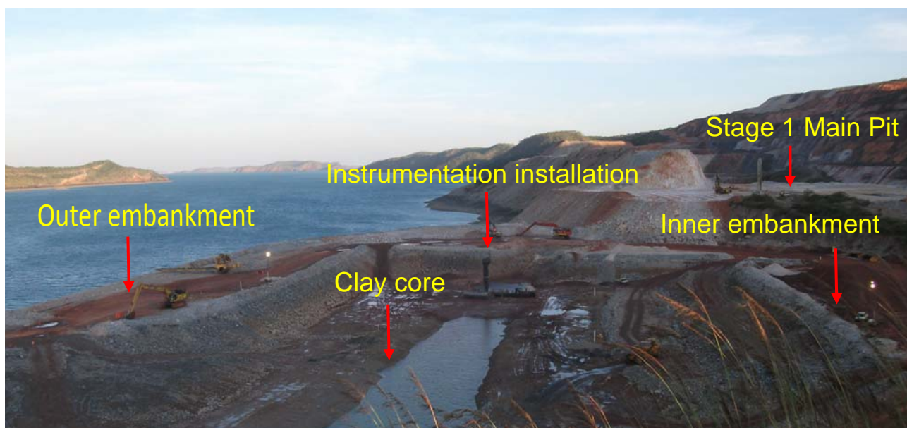
Figure 4 – Main pit seawall showing completed outer embankment looking west
