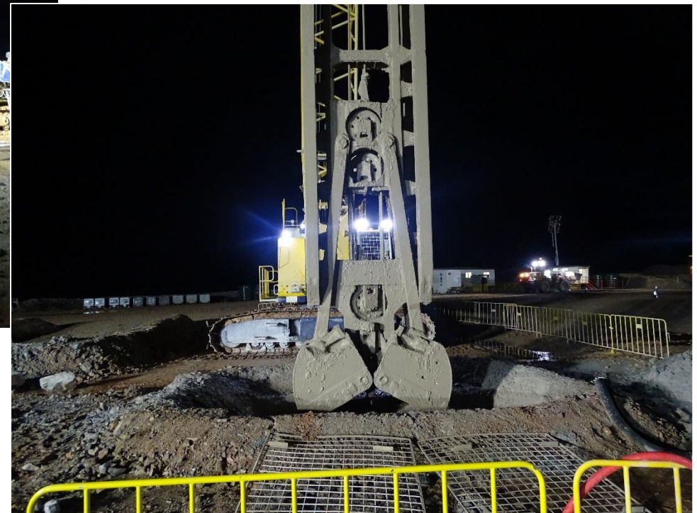
Panel excavation on night-shift, March 2018
