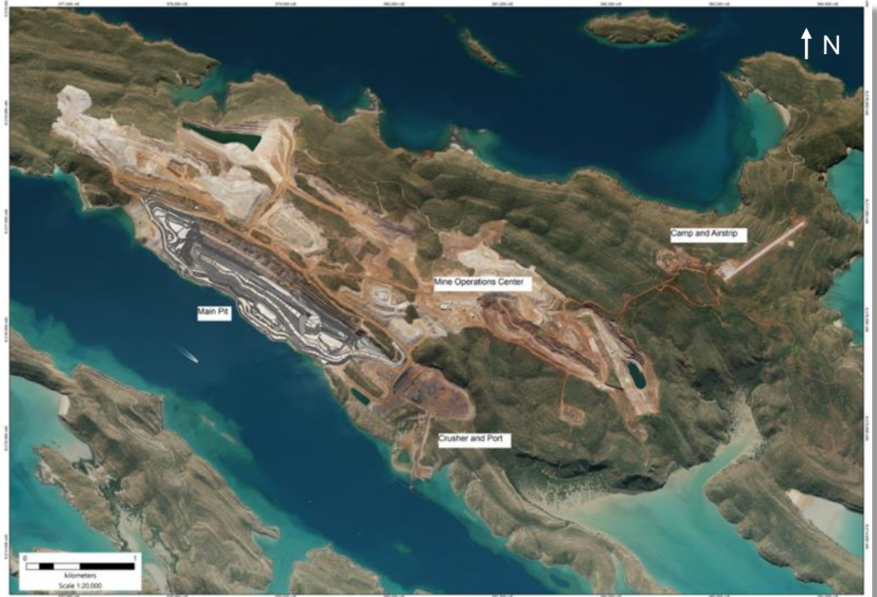
Koolan Island location and site layout showing Main Pit relative to existing site infrastructure, including crushing and port facilities, operations centre, accommodation camp and airstrip.
