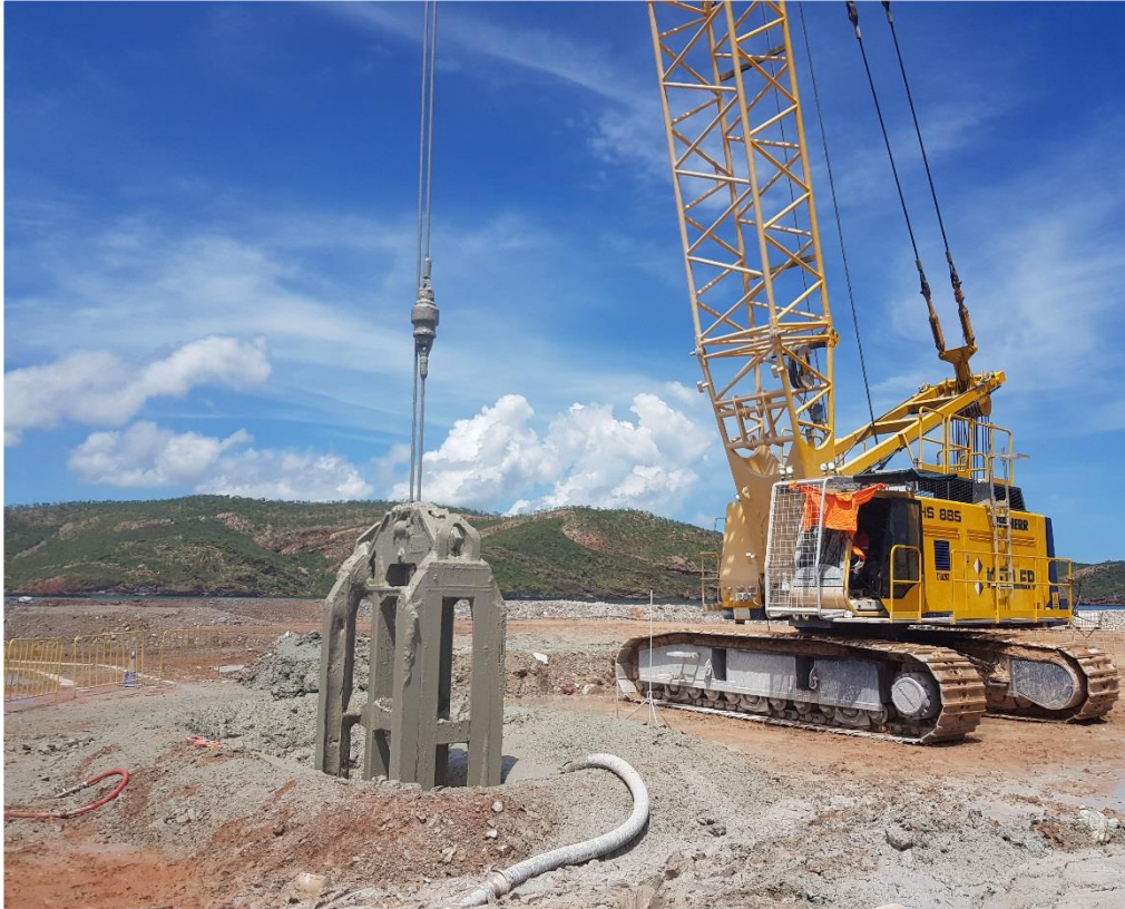
Grabber excavating seepage barrier panel March 2018
