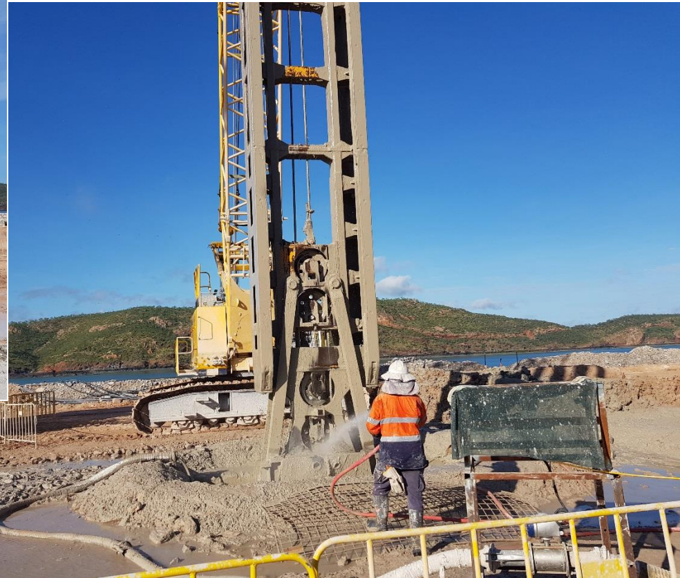
Panel excavation, March 2018
