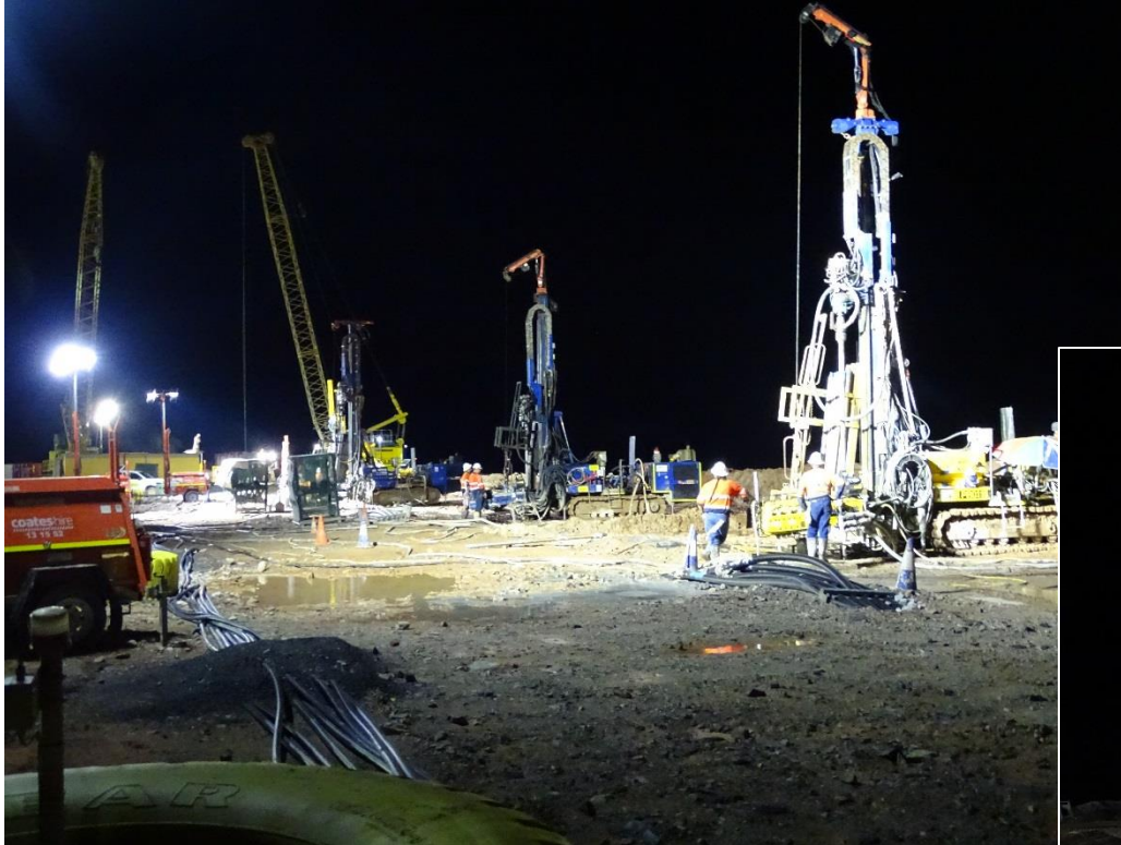
Grouting rigs working in central section of embankment, March 2018
