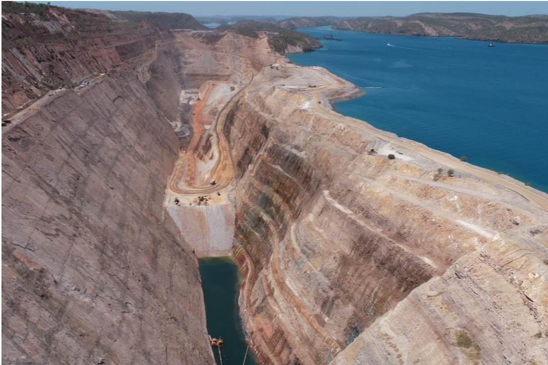
Figure 1: Koolan Island Main pit, looking east over the completed western end, showing the new central switchback and mine haul ramp, and the western water management sump, September 2024.
