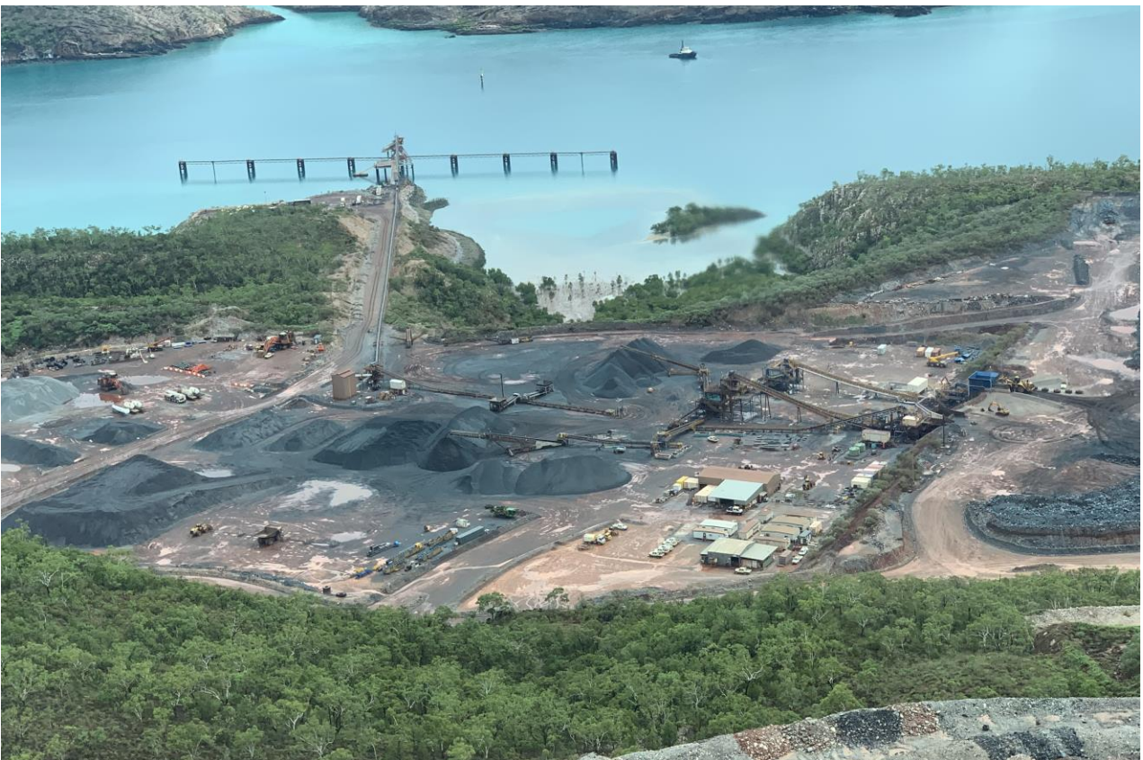
Figure 2: Koolan crushing and shiploading facilities, January 2022.
