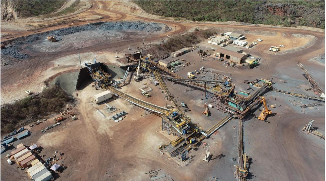
Figure 1: The upgraded Koolan Island crushing facility, showing the new ROM ore retaining wall, feed bin, jaw and cone crushers and screening circuits, December 2021.
