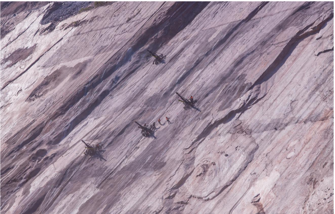
Figure 2: Main Pit upper footwall ground support work - installation of anchors, September 2021.
