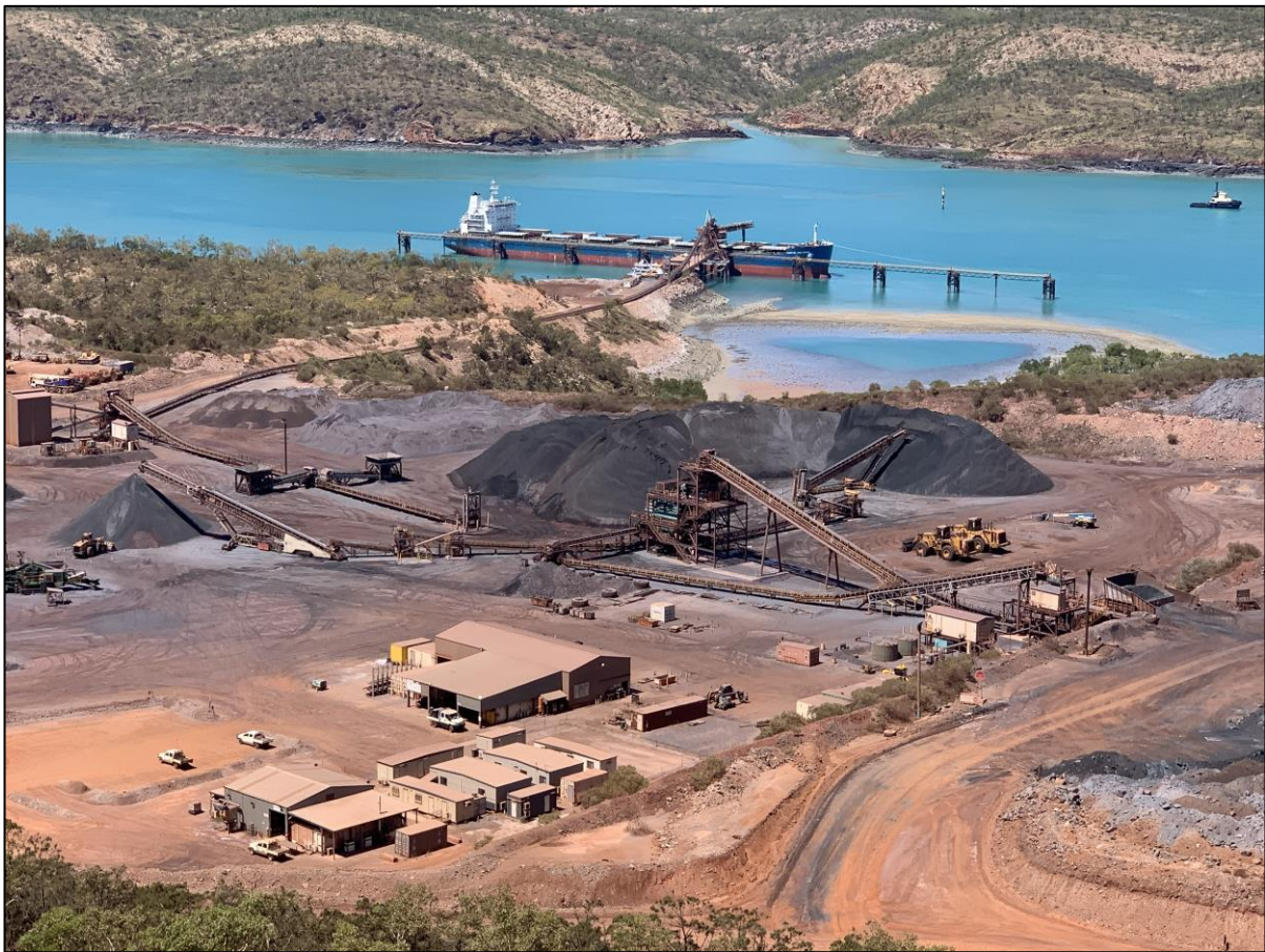
Figure 2: Koolan crushing plant, ore stockpile area, wharf and shiploading facilities, 24 September 2020.
