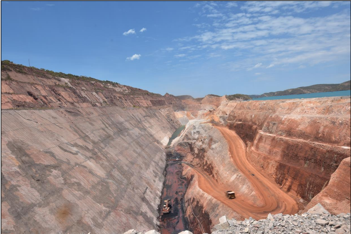
Figure 1: Koolan Main Pit, looking east, 3 October 2020.
