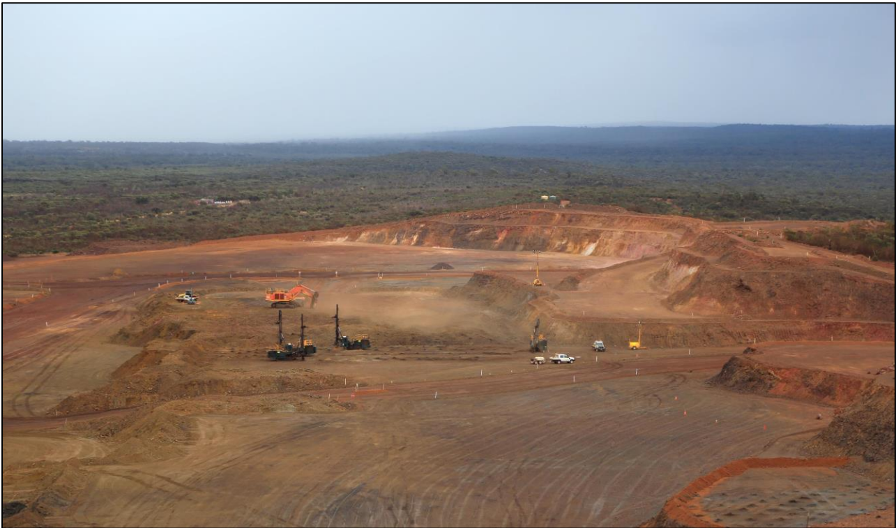
Figure 2: Mining in the Extension Hill open pit in August 2014, looking north.
