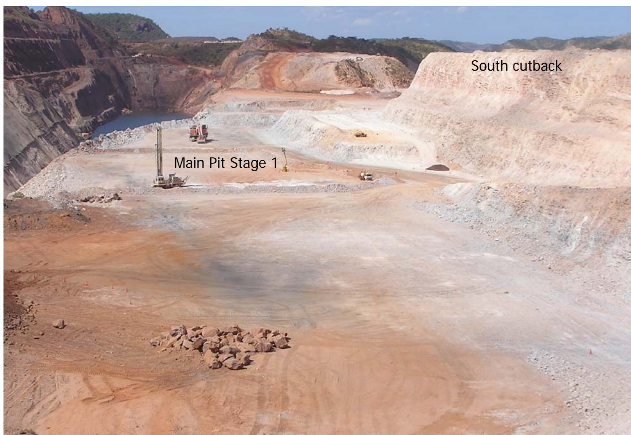
Figure 9 – Main Pit south wall cut back and Main Pit Stage 1 at the end of June 2011 looking east
