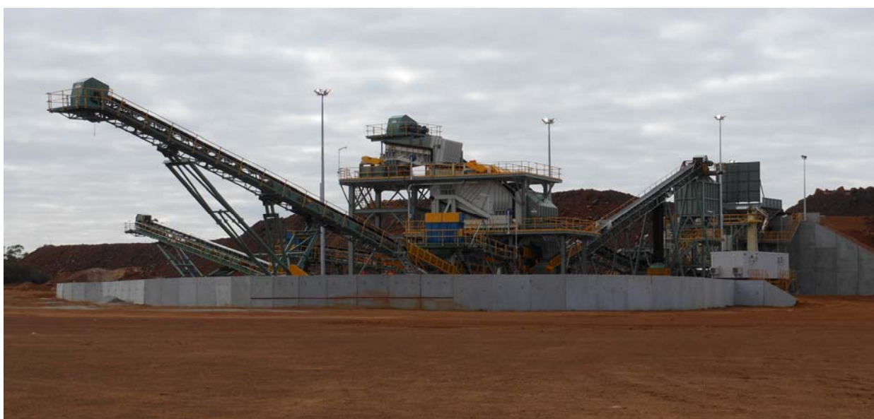
Figure 13 – Extension Hill crushing and screening plant
