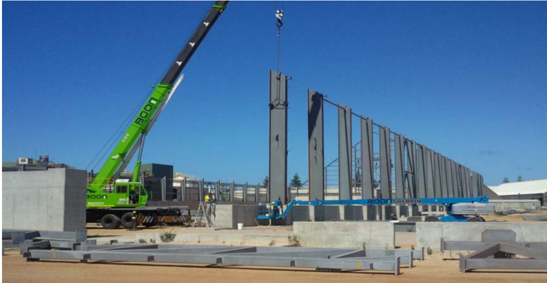
Figure 20 - Steel erection in progress – western side of new Berth 5 Storage Facility
