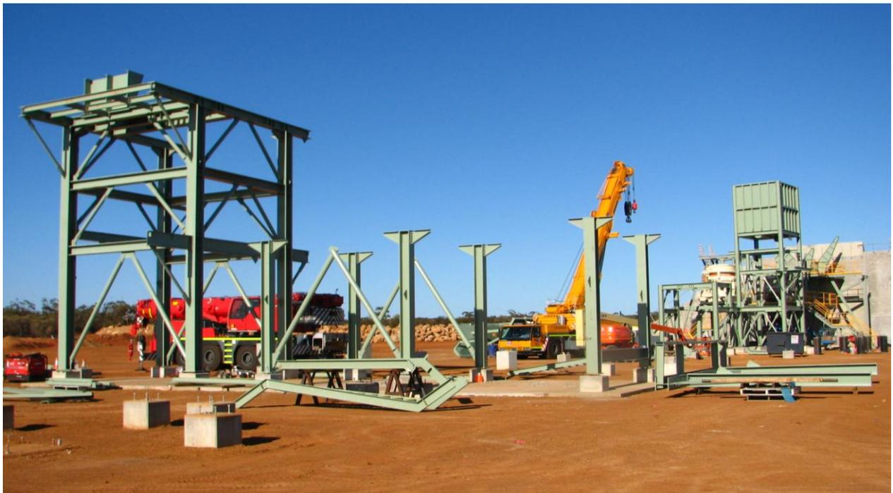
*Figure 14 – Crushing and screening plant under construction*
