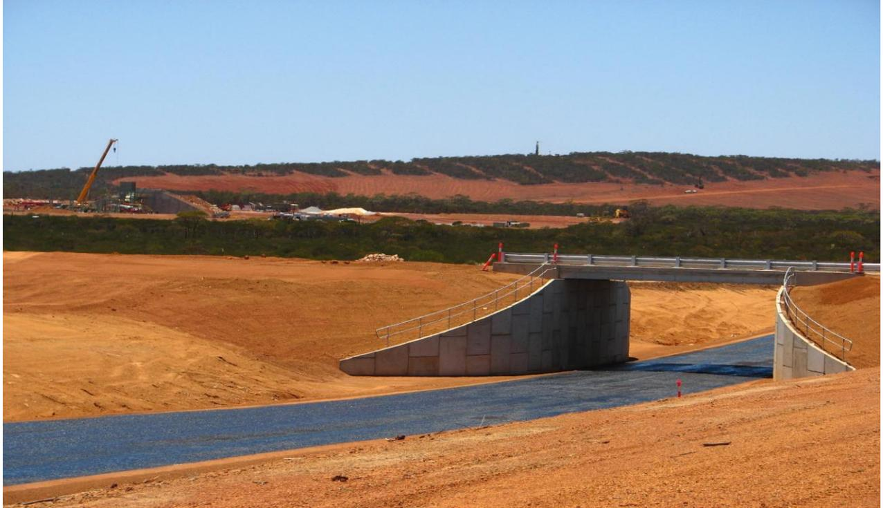
*Figure 13– Great Northern Highway Bridge with underpass primed & ready for sealing, crushing and screening plant and mine site in the back ground*
