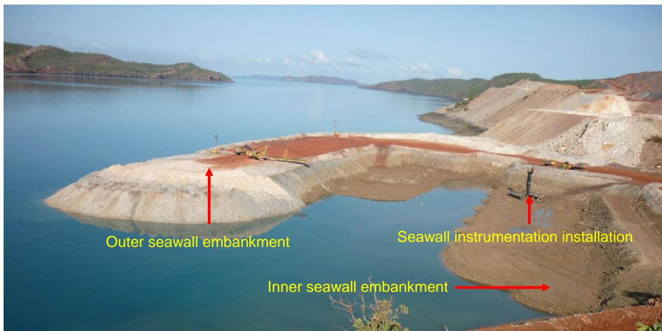
*Figure 9 – Seawall construction at the end of December 2010 looking west*
