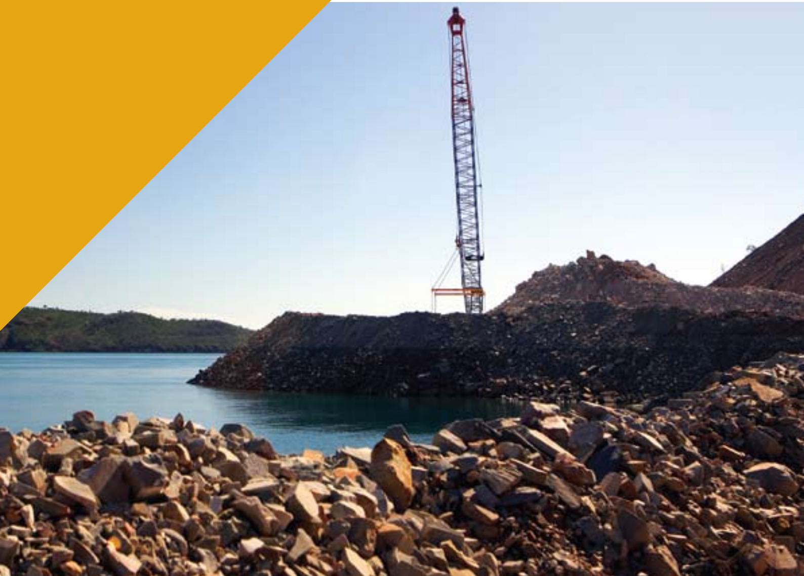
CONSTRUCTION OF THE SEAWALL ACROSS ARBITRATION COVE WILL FACILITATE MINING FROM THE KOOLAN ISLAND MAIN PIT.
